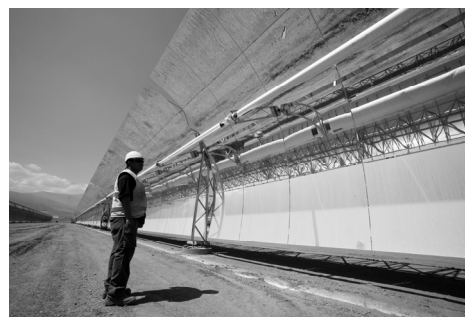
Fig. 4. Andasol powerplant in the south of Spain: mounting collectors
